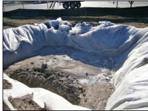
Plate 3.2 Concrete washout area
