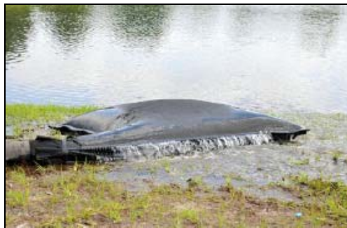
Plate 4.1 Silt Bag with water being pumped through
