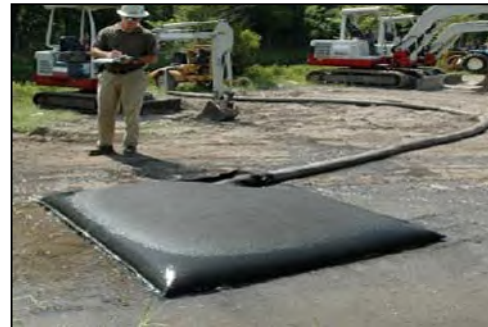
Plate 4.2 Silt Bag under inspection
