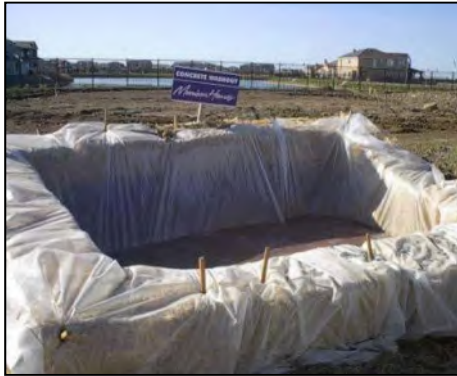
Plate 3.1 Concrete washout area
