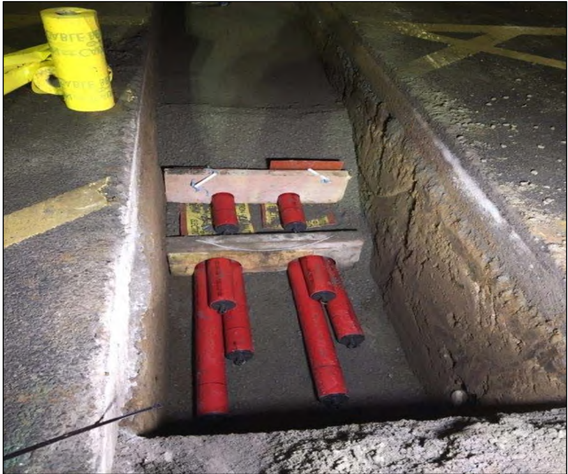
Plate 2.1 Typical Trench Views
